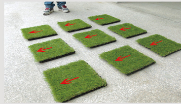
1. Put the grass tiles with all the grass yarn in the same direction.
