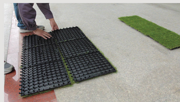
3. Lock in the strips one by one.
