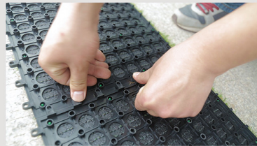
1. Put the grass tiles with all the grass yarn in the same direction.
