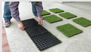
3. Lock in the strips one by one.
