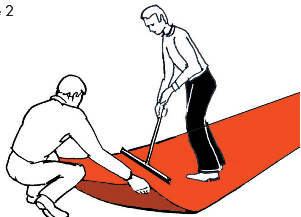
2. Squeegee out the bubbles while the other installer is holding the sheet up.
