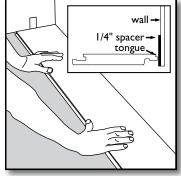
[1] Begin the installation in the left-hand corner. Place the plank a minimum of 1/4" from the left wall. Use the installation spacers throughout all perimeter areas to insure the correct expansion space is maintained.
